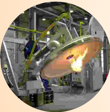
Ladle Pre Heater
